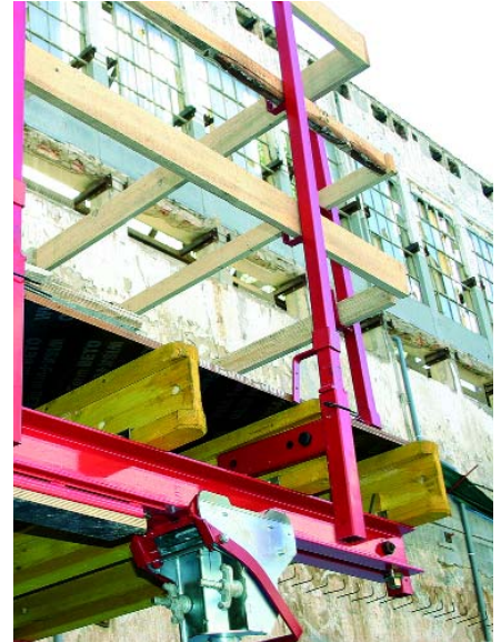
CONNECTOR AND GUARDRAILS FOR THE RAILING IN BOTH DIRECTIONS
