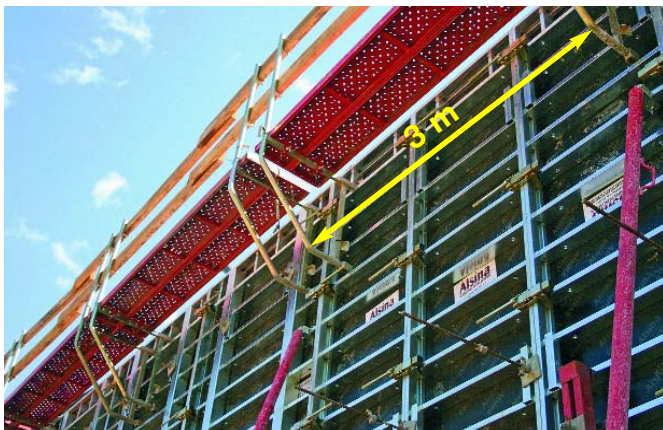
The Alisply Walkway Bracket with metal platform allows a maximum separation of 3 meters between platforms.
