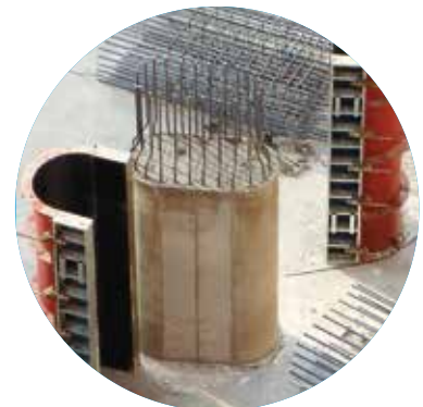
Detail of elliptic columns using a half pillar and Alisply Walls system.
