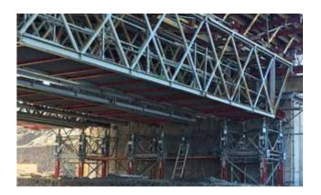
With a bending moment, up to 150Tn/m, the system can reach large spans up to 30m. There are some intermediate supports that can carry with the sharing forces making the system very flexible to solve many distributions.
