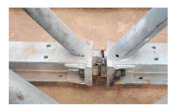
The Counter Bow system, easy and fast to do it thanks to the bolts of the bottom part of the structure. It allows to reach large spams with no permanent deformations in the superstructures achieving great results. The H33 Truss it is a reliable system designed to solve large spans for bridges solutions. It also allows to develop different applications as gangways and pier cap and other structural solutions.
