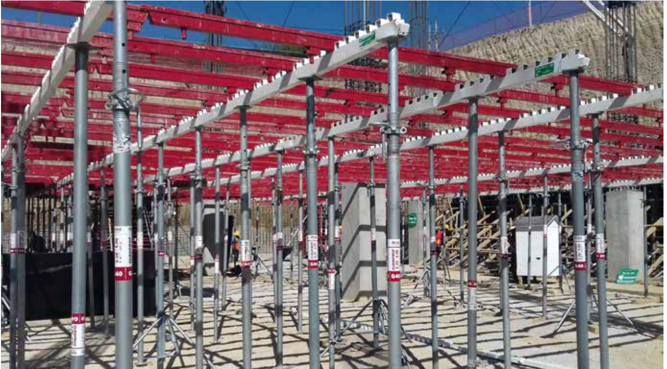
Office Park 4A Jalisco building, Mexico
