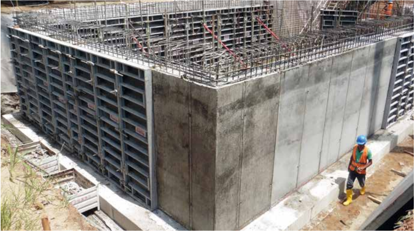
Hydraulic project in Asia
