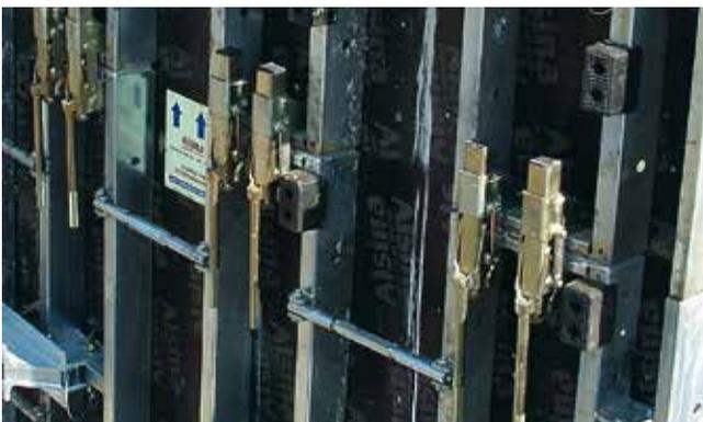
The Alisply GR-2 Clamp joins the modules of the Alisply Circular System horizontally and vertically. This operation can be carried out without tools. Because of the module's design, the clamp's position does not have to coincide with the position of the vertical posts. The GR-2 Clamp has a pressure regulator to adjust the joint strength.
