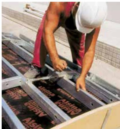
The panel includes the necessary elements to change the radius and special tools are not required.
