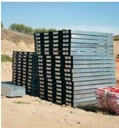
The Alisply Circular modules are preassembled at the warehouse, and only require to give it the correct radius at the job site.
