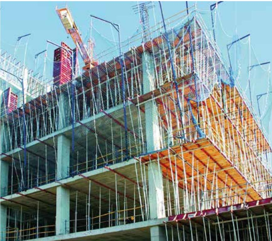
\*\* The 19'-8 1/4" (6 m) Post-shore can be used in either direction without affecting its performance.
