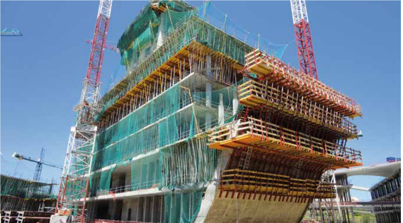
BBVA Bank Headquarters, Spain
