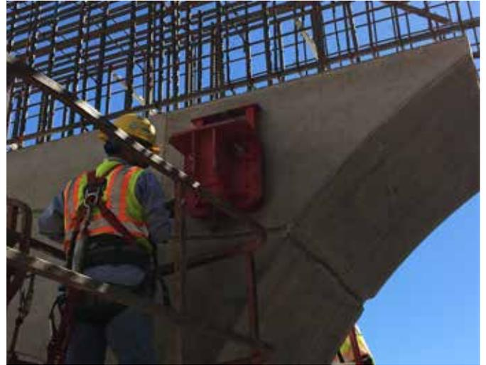
Placing brackets is easy and quick with our thru-bolts system. Alsina Engineering Department will provide the torque needed on the anchor bolts.
