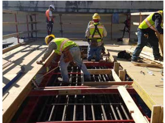
Once the form is on top of the brackets it is time to align side forms and close soffit panels. After working on final adjustments it is time to pour concrete.
