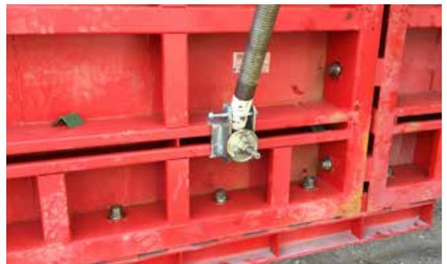
The Self Spanning System has a Multi-hole double channels that allows for one single panel size to fit in different cap widths (soffit and bulkhead).
