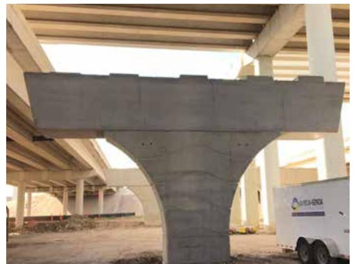
Once concrete strength has been reached, soffit needs to be opened and stripping can be made in one single crane movement.
