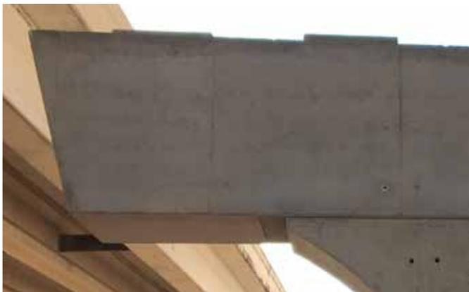
Rustication, Chamfers and Form liners can be attached to the form face. The Steel face sheet provides a great finish, reducing finishing costs.
