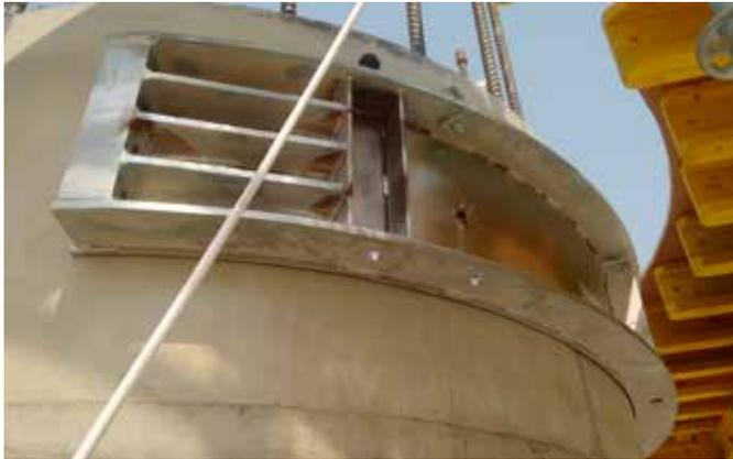
Friction collar is a temporary support that transfer the vertical load to the concrete columns by friction between concrete and collar. This solution transfer the loads to the concrete column with no need of anchors.
