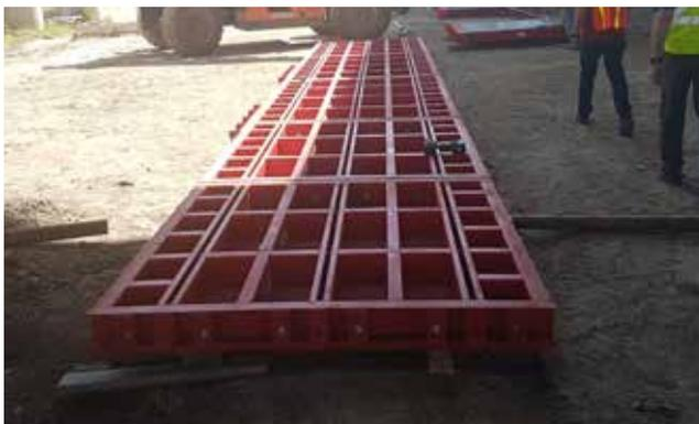
The Self-Spanning System has 16 panels sizes with heights up to 10' and lengths up to 12'.
