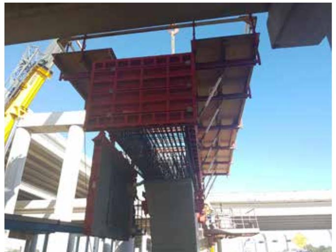
With one single crane movement, form is placed on top of the brackets.
