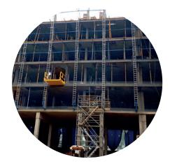
No interference with the installation of auxiliary equipment like unloading platforms, access ladders, etc.
