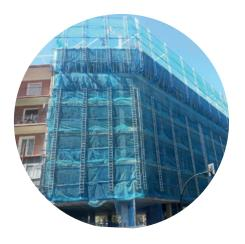
Net system with U shape, which adding an additional internal netting, it can provide full height containment.
