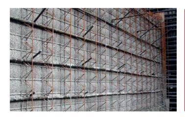
Stremaform® formwork elements for working joints from MAX FRANK divide large structural components into individual concreting sections. The prefabricated elements are used as permanent formwork in floor slabs, ceilings and walls.
