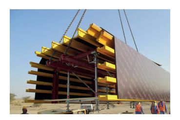
Plywood board with 120 g/m $^2$  phenolic surface coating. Its exclusively birch composition generates very high mechanical strength and makes it possible to reuse it many times.
